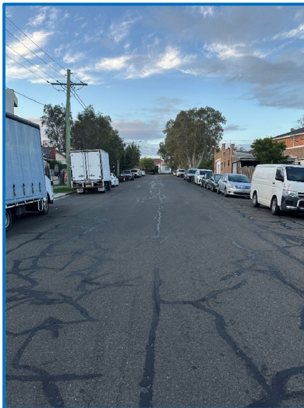
Figure 4a: Kent Street: Looking West to the Intersection
